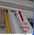
until a good seal is achieved. To prevent the screen door from being closed too far and potentially damaging the Bug Warden, a stop washer is installed. Hold the washer in the top of the screen door sliding rail and mark drill hole with pencil
